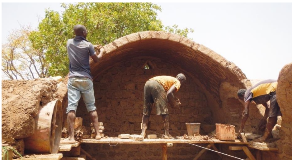
A Nubian Vault construction site
