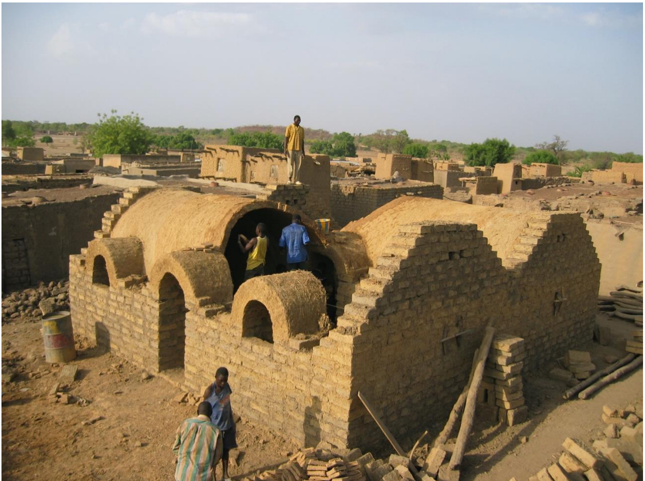
A NV construction site
